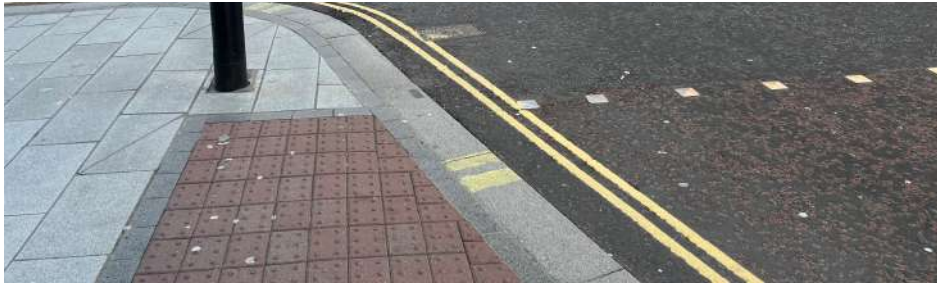
Example of diagonal crossing point
