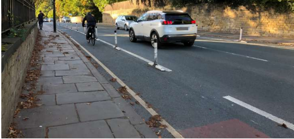
*Example of wands and orcas currently in place on parts of A660.
